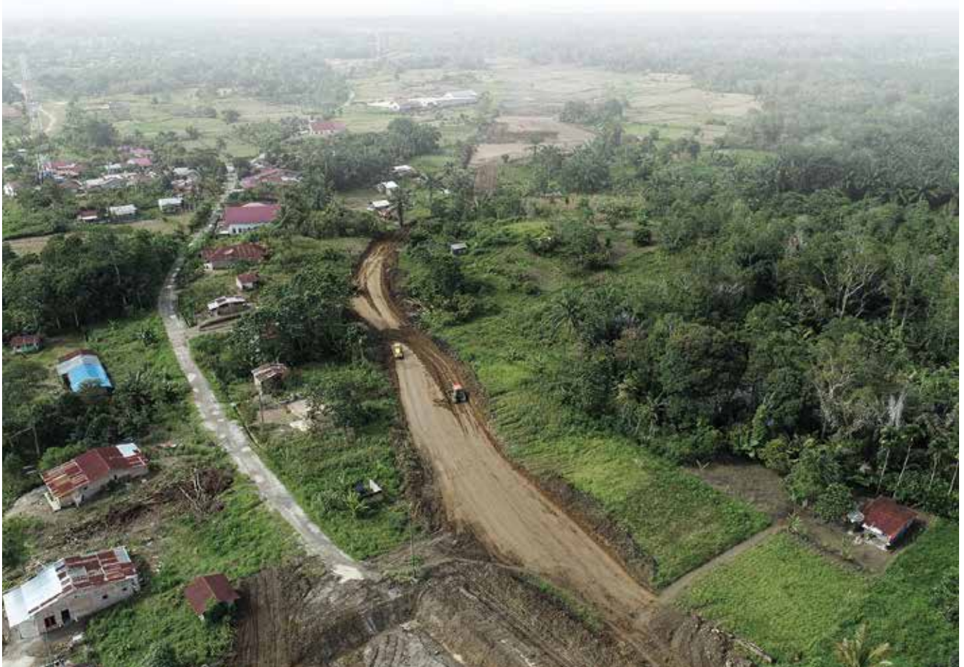
Clearing lahan Jalan Tol Kuala Tanjung-Tebing Tinggi-Parapat, Sumatera Utara.
